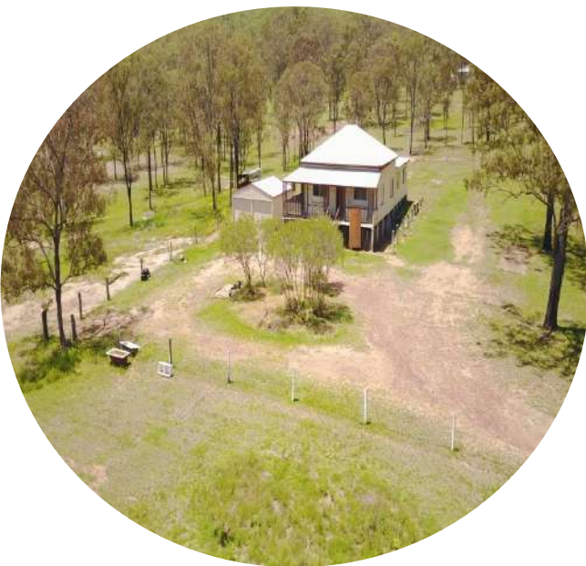
153 Access Rd, Rosevale
